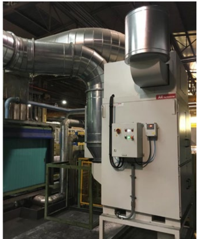
AR 10.000 installation on SACMA automatic presses
